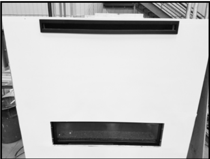
Figure 6 Vent Cover Installed
